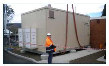
Pier footings were nominated and installed as well as a concrete foundation for the emergency plant and supporting conduit system.
