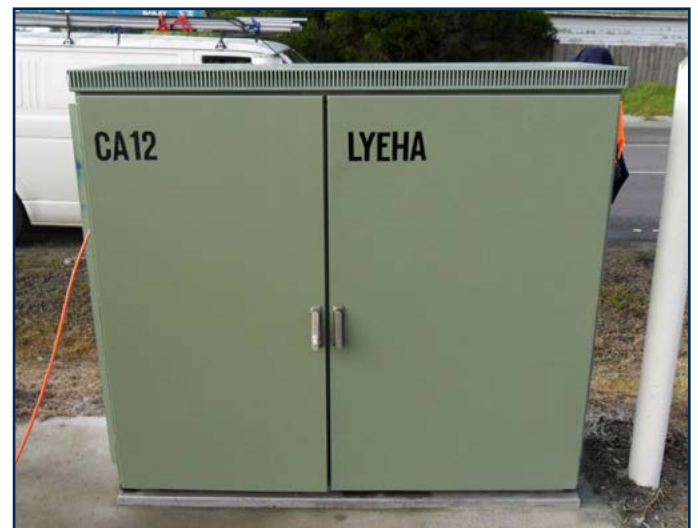
4. Work completed with new doors and straightened frame
