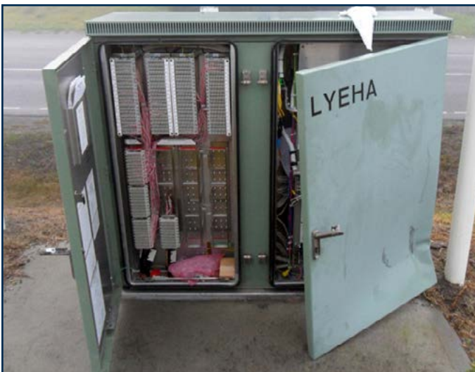
3. Repair included refitted doors, instruction panels and DA numbering
